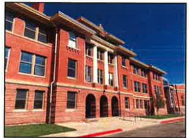
High School Building B
