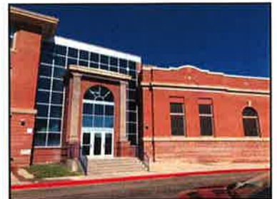
Atrium connecting 1922 Addition
