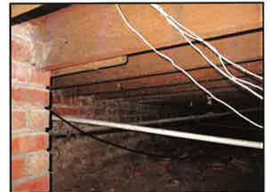
Joists seem to be in good condition
