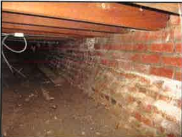
Interior crawlspace showing below grade walls and floor joists
