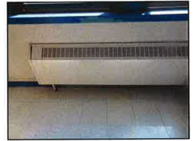
The classrooms in the 1911 building are conditioned by hot water baseboard convectors. None of the rooms have any cooling or mechanical ventilation.
