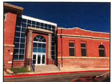
Atrium connecting 1922 Addition
