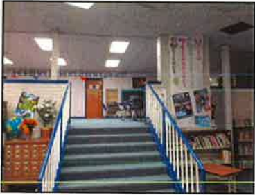
Typical T8 Lighting Fixtures
