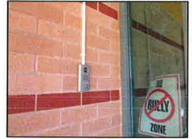
Secure main entrance
