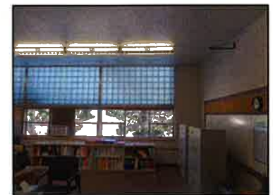
The classrooms in the 1964 Park Street addition have a large amount of glass block
