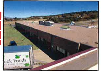
East Wing Classrooms
