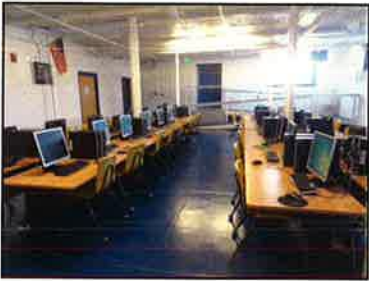
Despite the 1993 electrical upgrade, many of the classrooms still have an inadequate number of outlets
