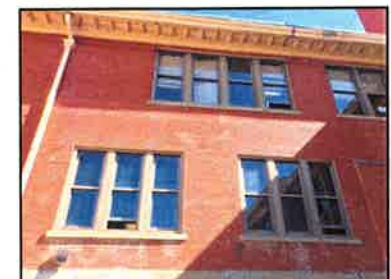
Windows are typically propped open for outdoor air to combat comfort issues
