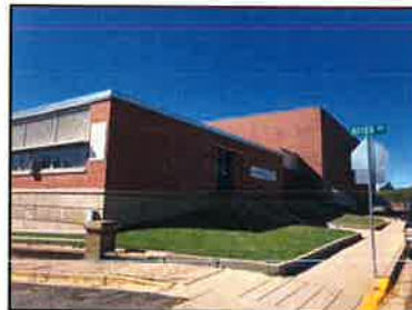
Park Street Main Entrance
