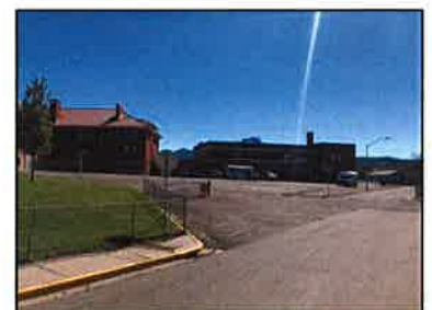
East Parking Lot exiting onto Hillside or Willow St.'s
