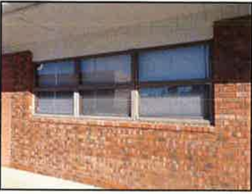
The 1964 wing has aluminum framed windows that are in serviceable condition.
