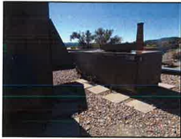
The cafeteria and gymnasium in the 1993 building are conditioned by rooftop furnaces. They are over twenty years old and need to be replaced.
