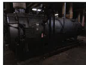
The large hot water boilers serving the building are 40 years old and are extremely inefficient. They need to be replaced with a smaller, more efficient boiler plant that is easier to maintain.
